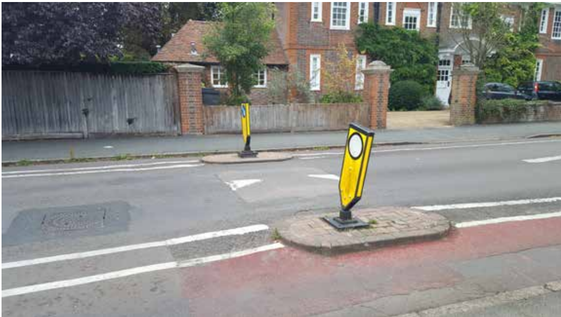
Semi-diverter narrowing roadway to one lane
