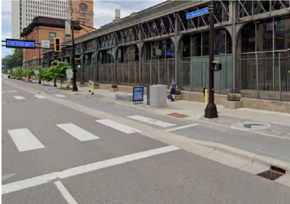
Curb height protected bike lanes on S. Washington Ave in downtown Minneapolis
