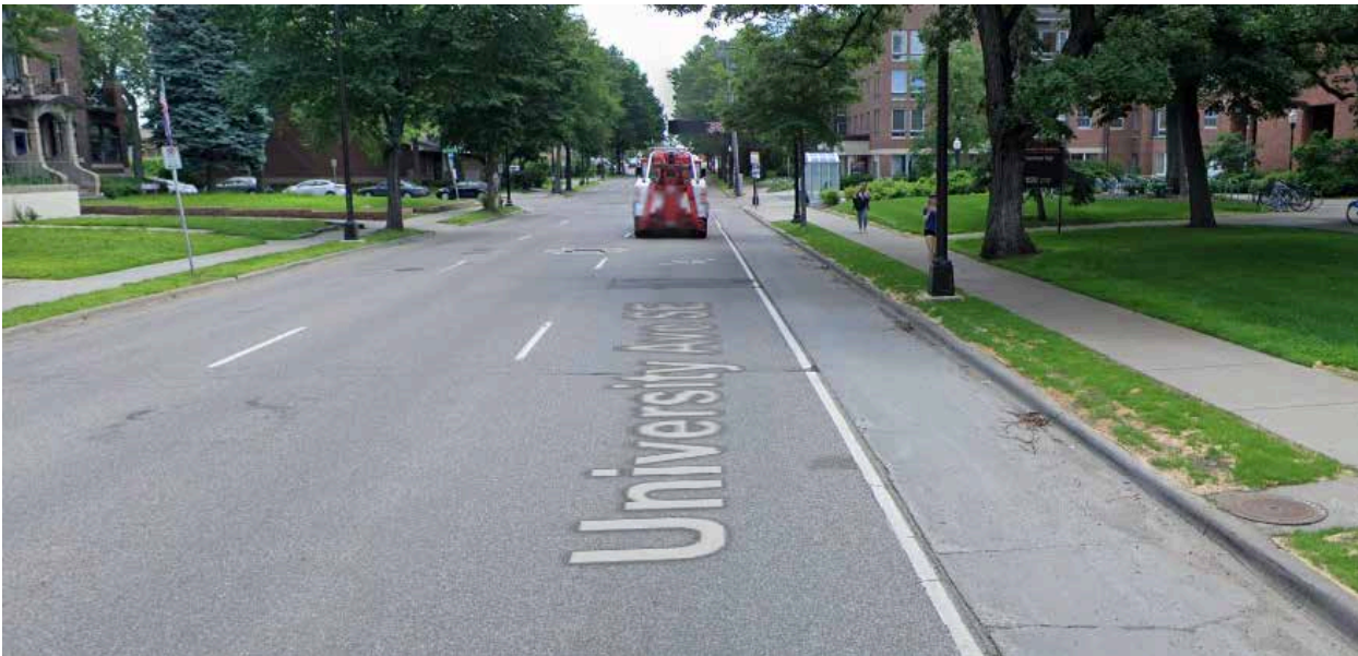
University Ave SE: Current conditions with three vehicle lanes and an unprotected gutter-pan bike lane
